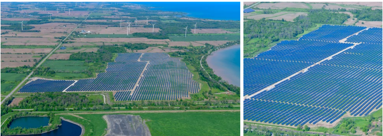
Nanticoke Solar Project
