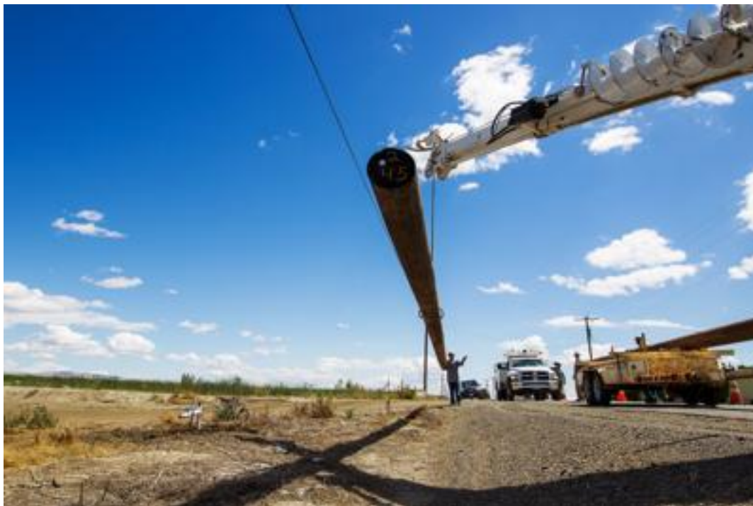
Figure 24. Yakama Power Crews Place Utility Poles
