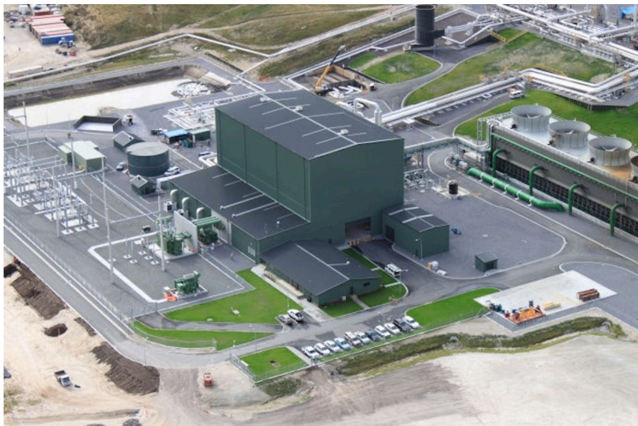
Figure 19. Nga Awa Purua Geothermal Power Station
