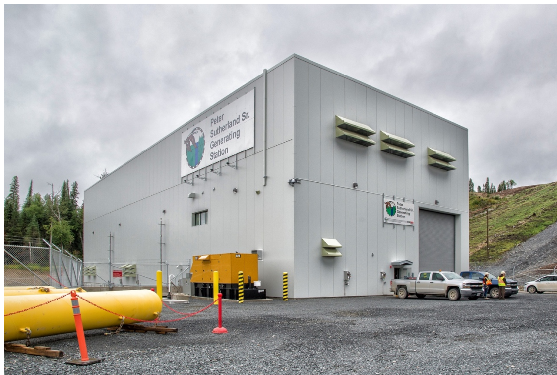
Figure 22. Coral Rapids Powerhouse
